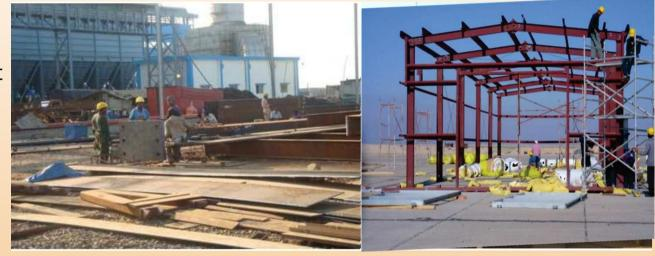
No welding is required at site and so it can be erected at site where electricity is not available. Most Effective as These sheds can be resold.
